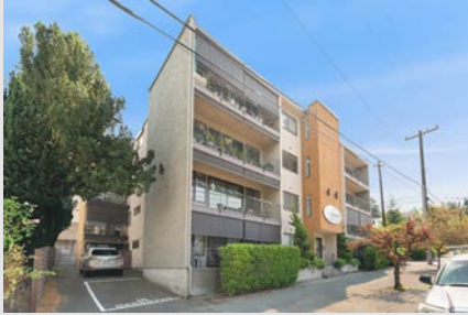
Haven Apartments 7130 California Court SW
