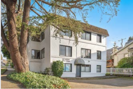
Eastlake Office Building 207 E Edgar St, Seattle, WA 98102
